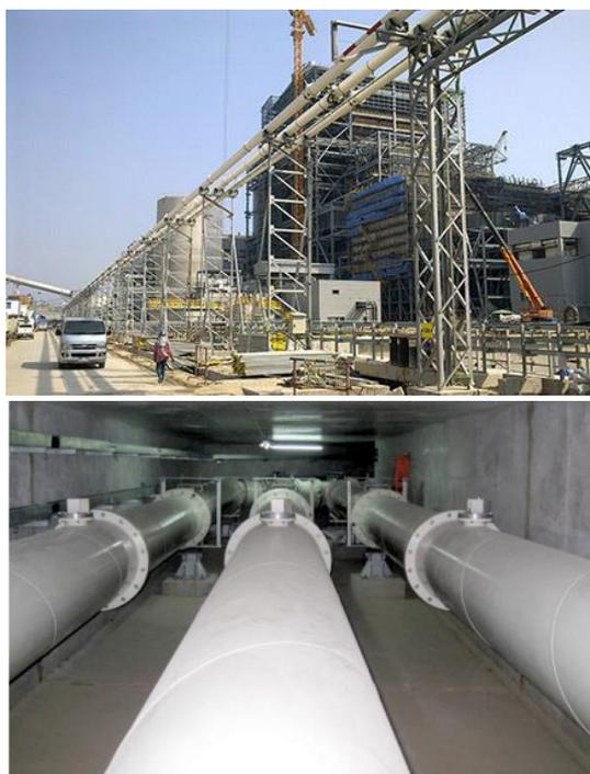
*Figure 1 - GIL installations in power stations; above ground (left), and underground (right)*
