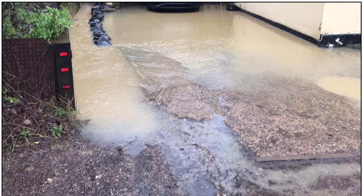
Image 3 - Watercourse overflowing onto Tuddenham Lane
