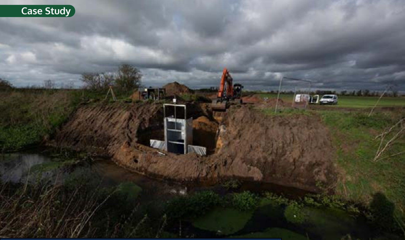
Sluice and pipe under drove in construction at Lakenheath Fen
