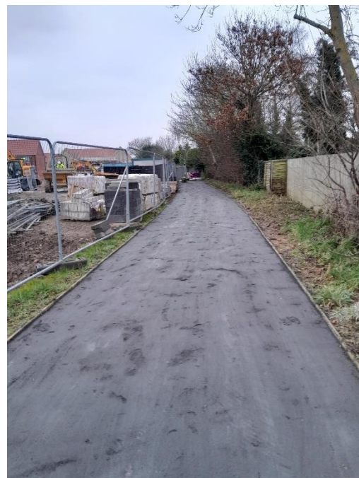
Resurfaced footpath leading east
