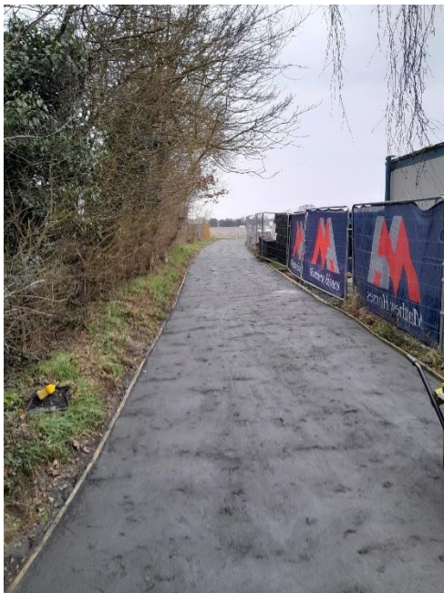
Resurfaced footpath leading west
