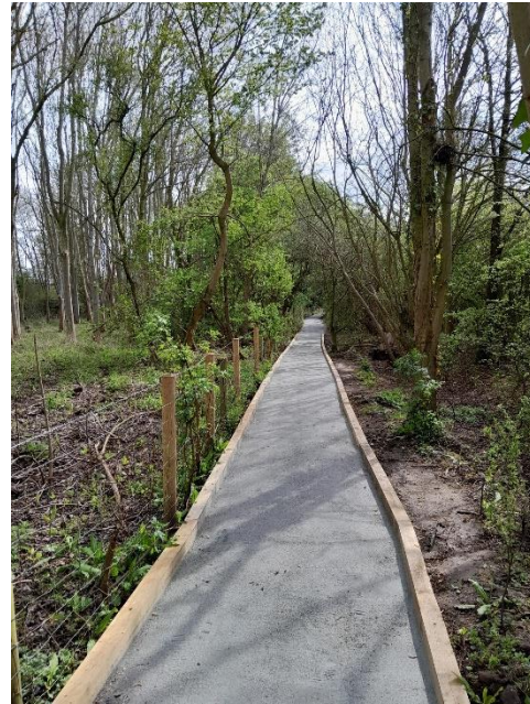
Footpath with completed new surface
