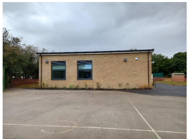
New classroom block
