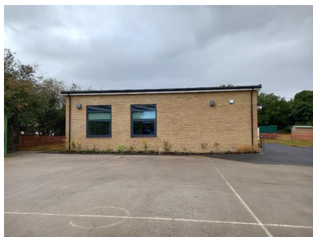
New Primary School Block, Martlesham
