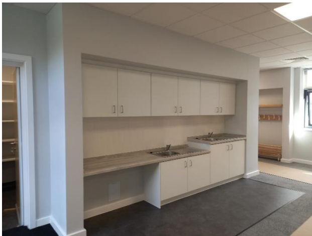
Utility area in new block
