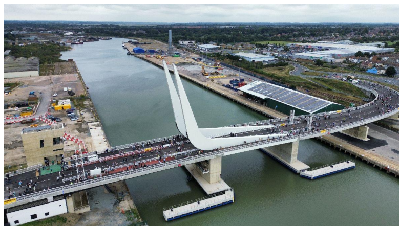
Gull Wing Bridge, Lowestoft
