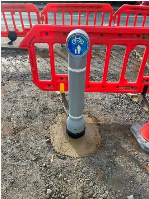
Footway under construction
