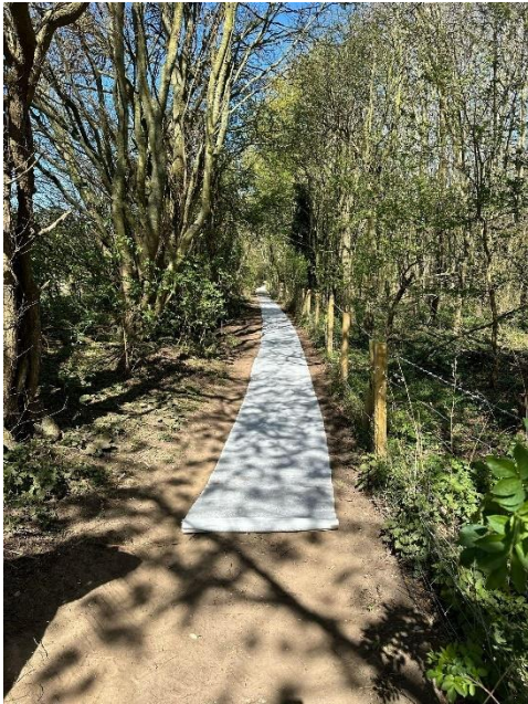
New surface under construction
