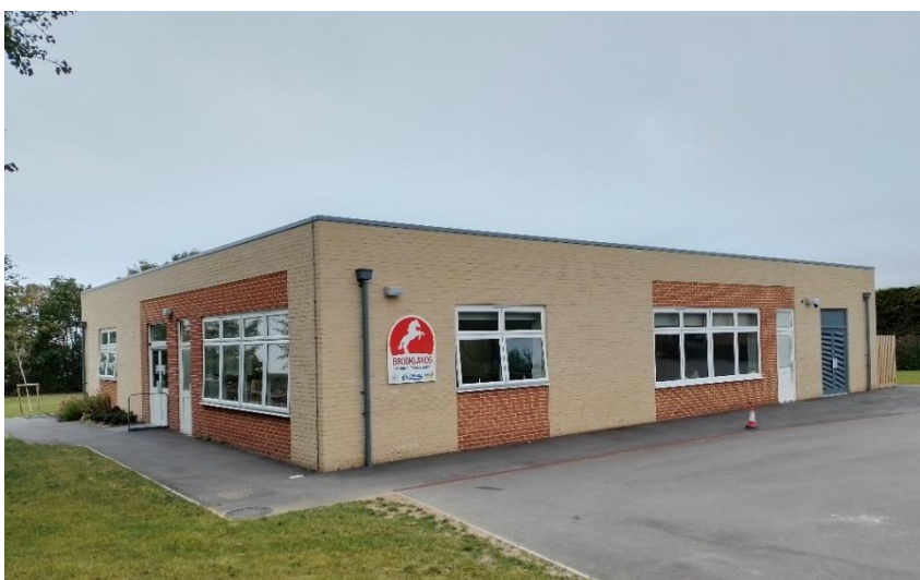
Brantham, Brooklands Primary School expansion
