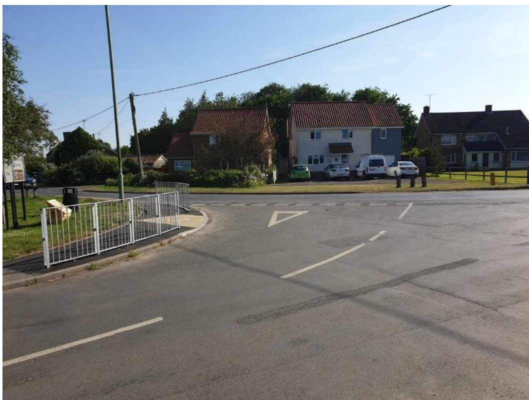
Framlingham, East Suffolk – Pembroke Road Junction Improvements
