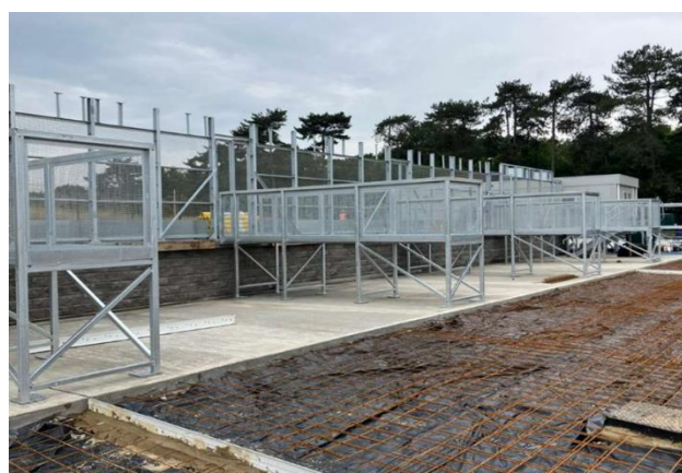
Foxhall Recycling Centre - same level recycling access
