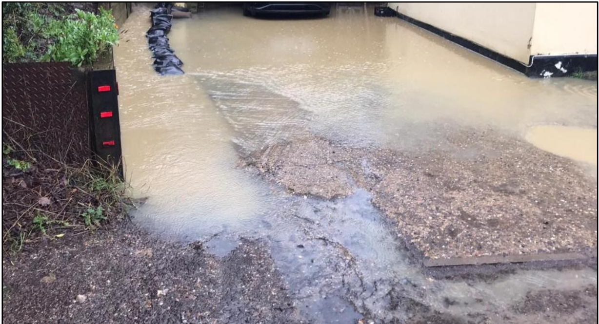
Image 3 - Watercourse overflowing onto Tuddenham Lane
