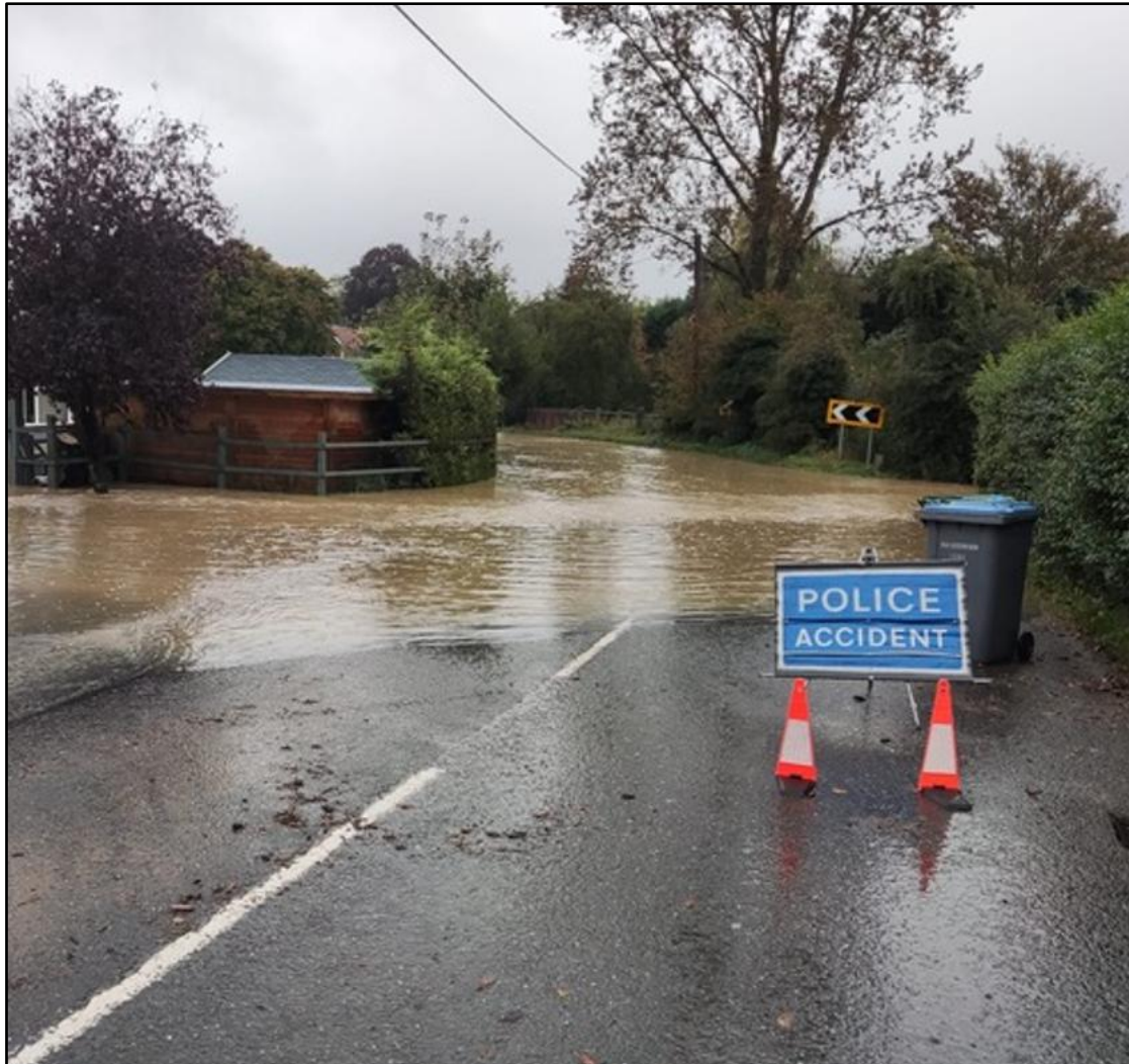
Image 1 - Looking north towards River Fynn road bridge
