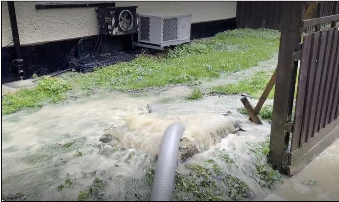
Image 6 - Surcharging manhole outside Barley Mow public house
