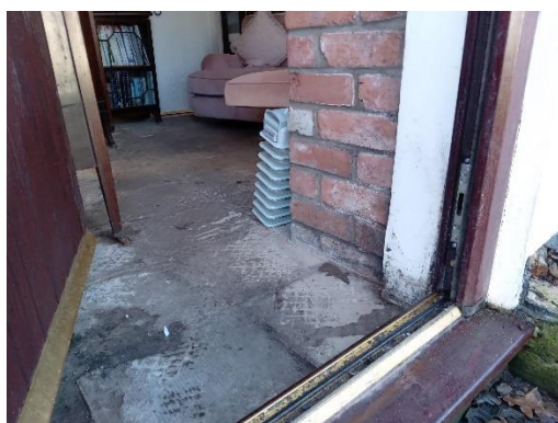
View into front room from outside front door, showing extent of where all floor coverings including floor tiles have lifted (and had to be removed) because of repeated internal flooding.
