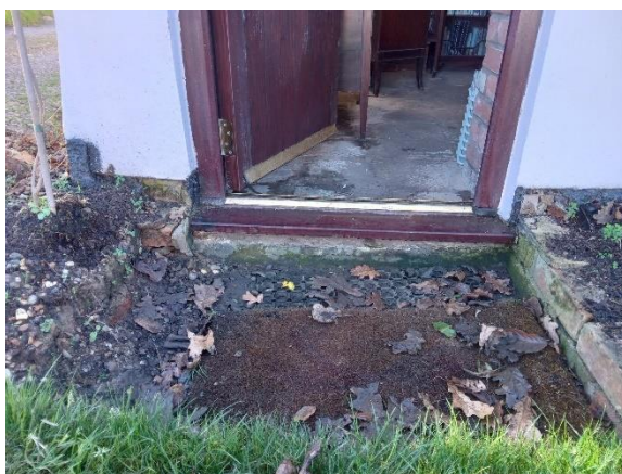
Front entrance to property, showing external step down at threshold
