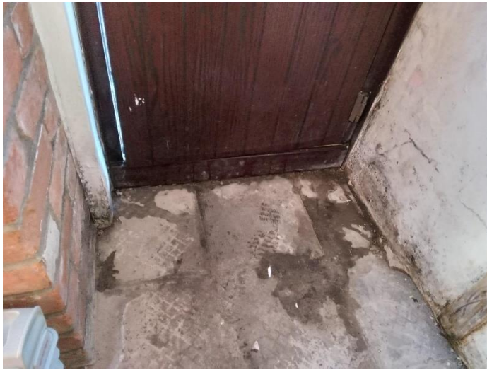
Front door, viewed from inside, floor tiles lifted (due to flood) and removed.
