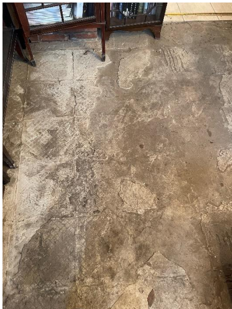
View of floor of front ground floor room showing water saturation of the foundation level.
