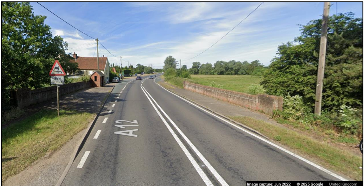
Image 2 - A12 road bridge over the river Ore
