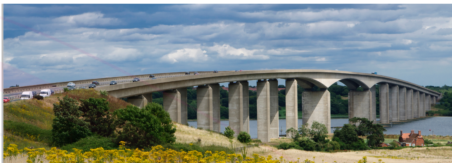
The Orwell Bridge in Ipswich
