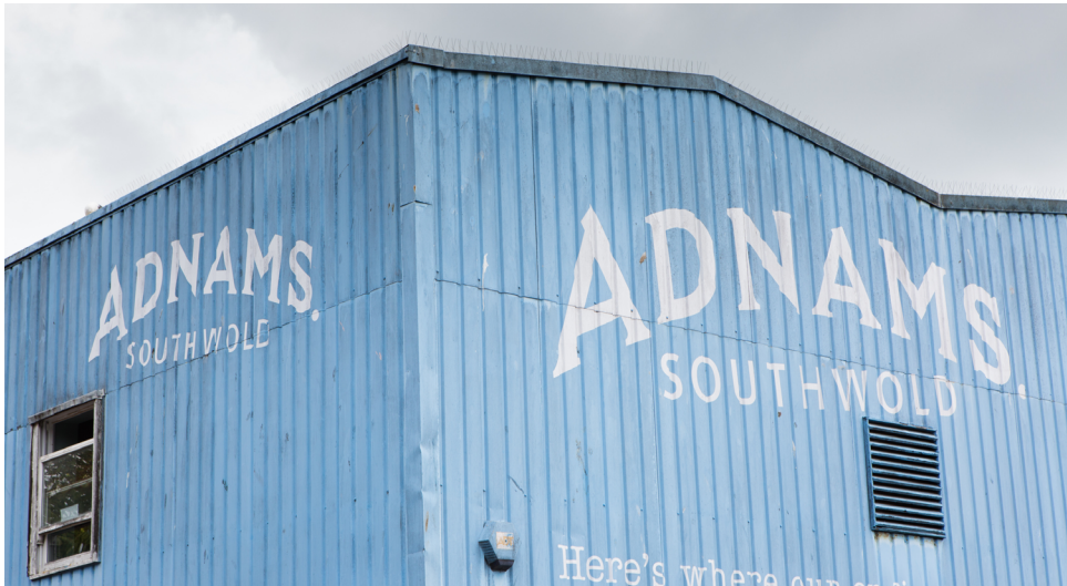
The Adnams Headquarters in Southwold
