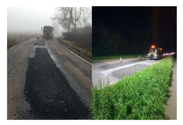
For the urban areas we have commenced a trial using RoadMender Elastomac Patching. Elastomac works on both asphalt and concrete roads and is designed for repairs to cracks, joints, potholes, patching, surrounds to iron work, fretting, wheel rutting, kerb channels and speed ramps. This trial commenced in Mid-March 2024 and will be reviewed after the first month, if successful this will become another product available to us to support our network.
