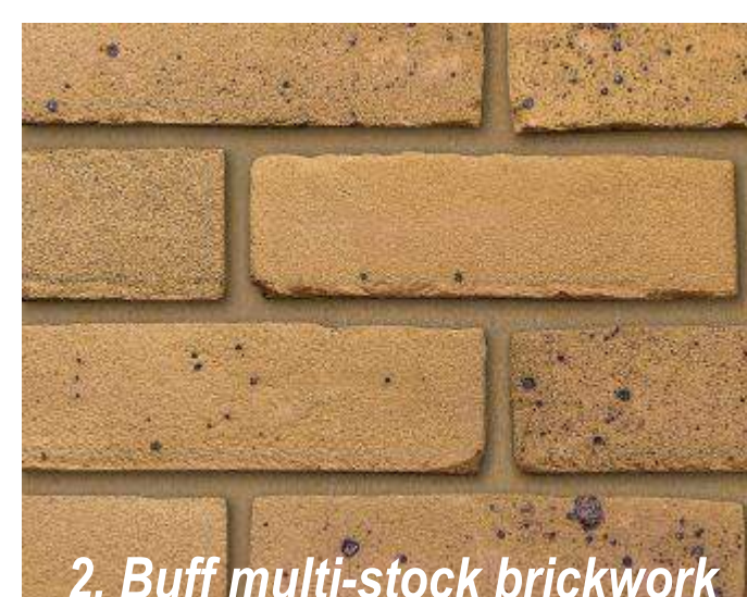
2. Buff multi-stock brickwork
