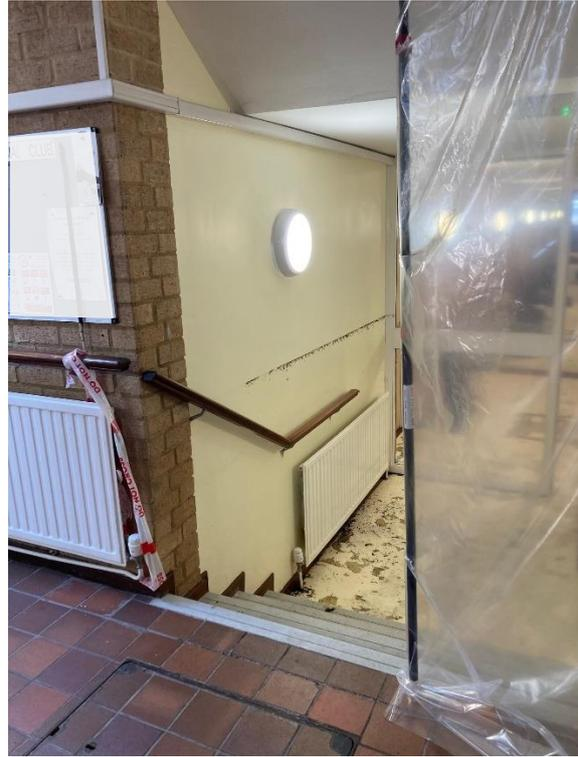
Depth of flooding internally within the corridor serving the retirement flats, see watermark
