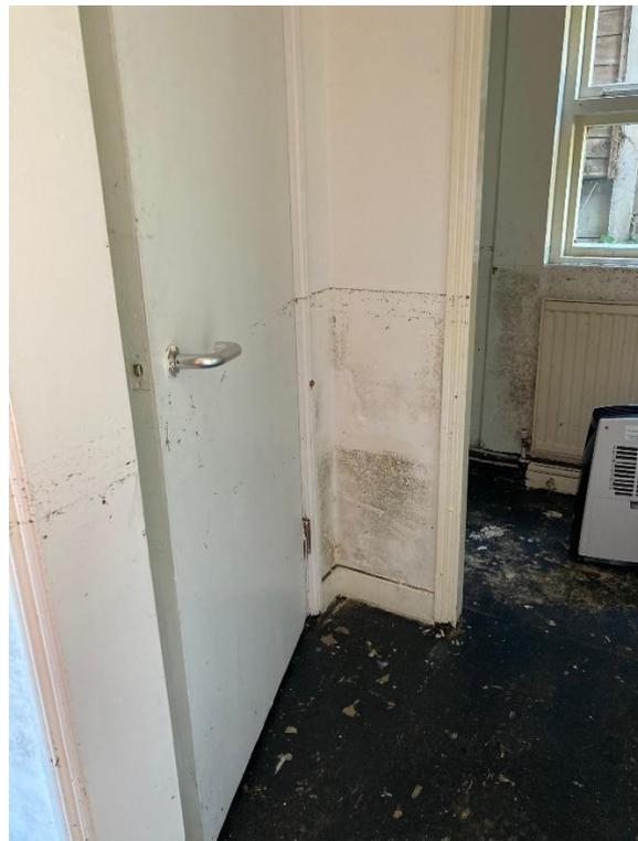
Depth of flooding internally within 'basement' floor of semidetached property, see watermark
