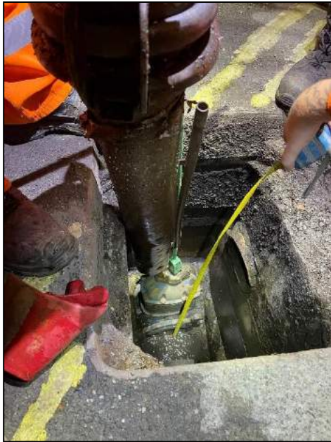
Inspection of the surface water drainage penstock at Fen Lane, Beccles in July 2021.
