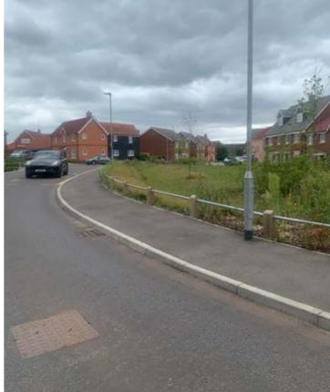
Asphalt concrete should be used as the surface finish for the majority of footways and cycletracks to be adopted by the highway authority. Coloured surfacing can be used by designers to clearly delineate features within streets and identify segregated cycle infrastructure. Coloured surfacing may be particularly useful in the following situations:
