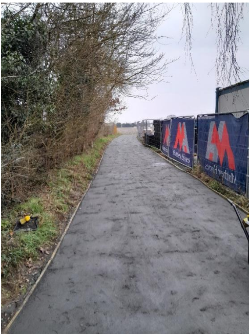
Resurfaced footpath leading west
