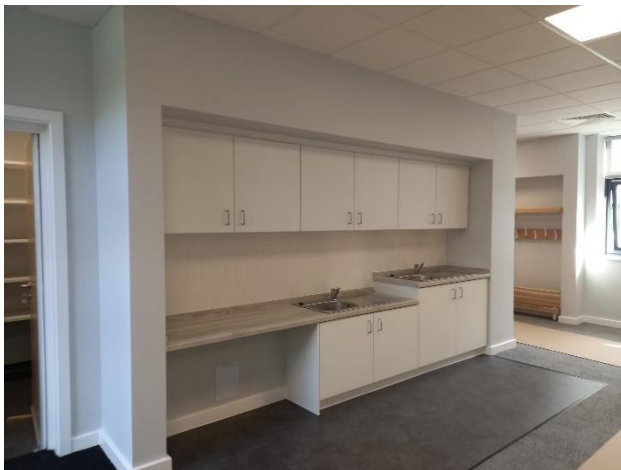
Utility area in new block
