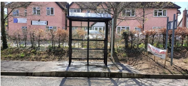
New Bus Shelter, DDA kerbs and hardstanding at Village Sign (opp)
