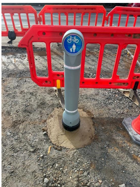
Footway under construction
