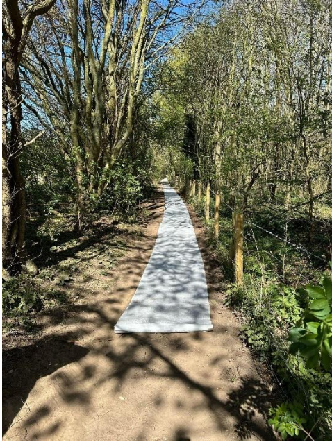
New surface under construction
