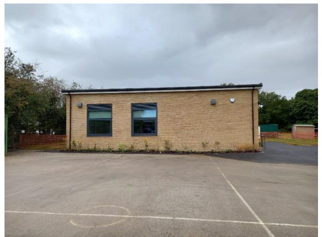
New classroom block
