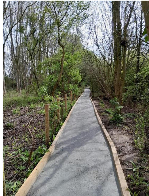
Footpath with completed new surface
