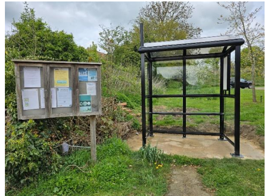
New Bus Shelter at Village Sign stop
