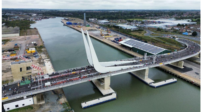
Gull Wing Bridge, Lowestoft
