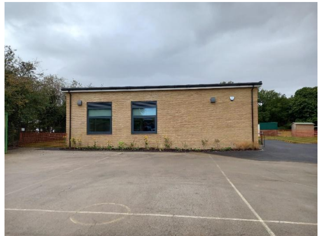
New Primary School Block, Martlesham
