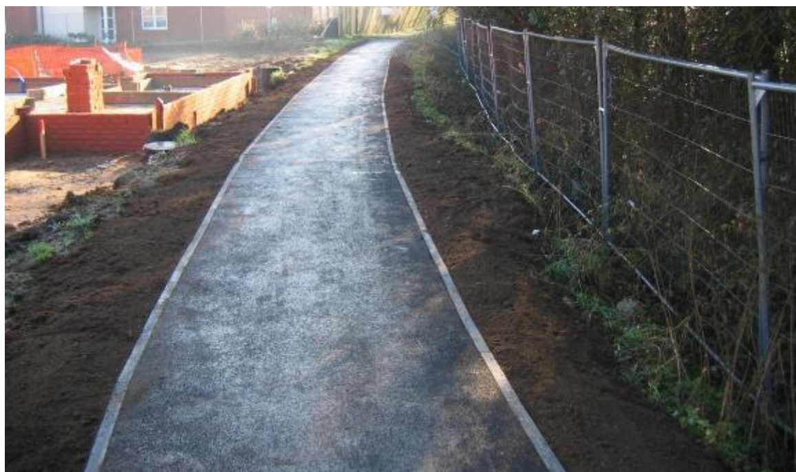
Photo of footpath improvement scheme, Stowmarket
