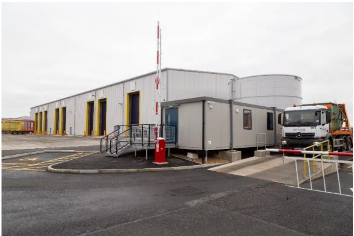
Photo of West Suffolk Operational Hub
