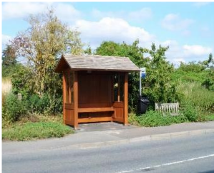
Photo of bus shelter, Newton
