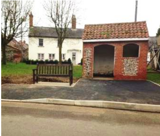
Photo of bus shelter, Gazeley
