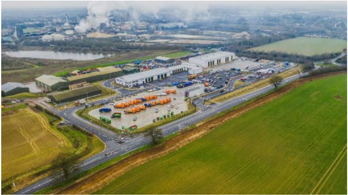
Photo of West Suffolk Operational Hub
