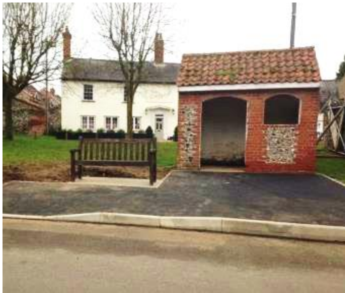
Photo of bus shelter, Gazeley
