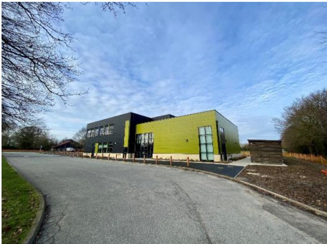
Photo of Stowupland High School Expansion
