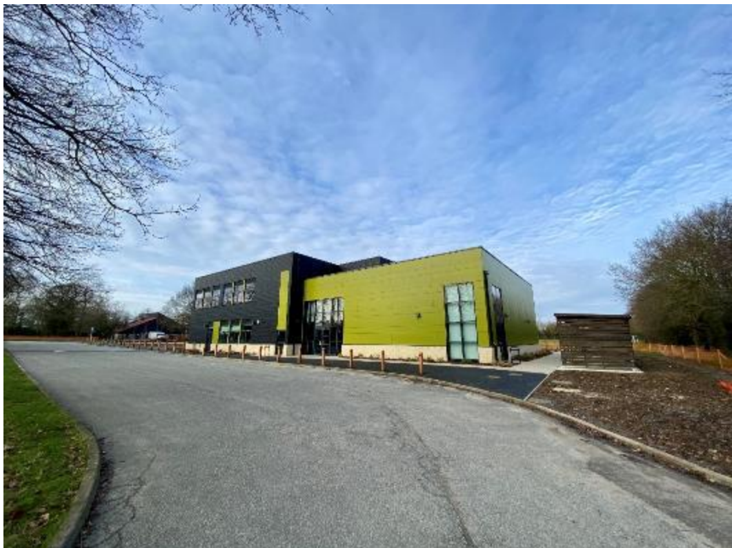
Photo of Stowupland High School Expansion
