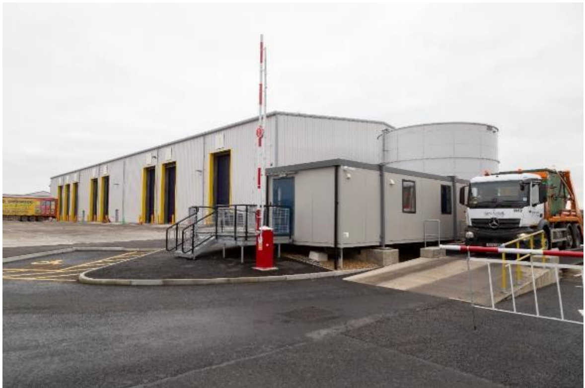
Photo of West Suffolk Operational Hub
