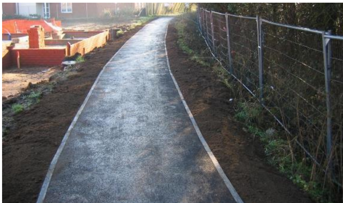
Photo of footpath improvement scheme, Stowmarket
