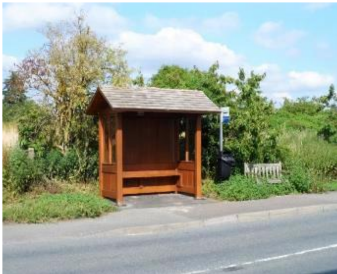
Photo of bus shelter, Newton
