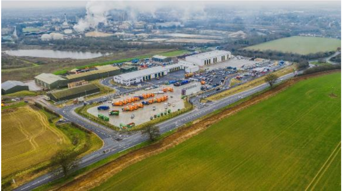
Photo of West Suffolk Operational Hub
