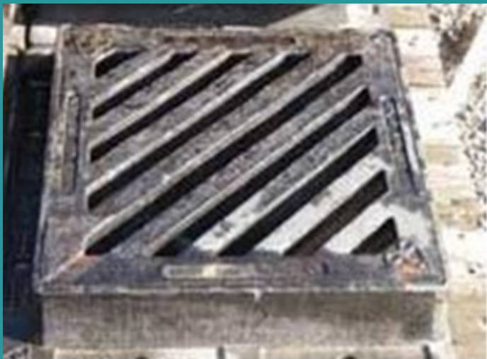
A drain grating and frame
