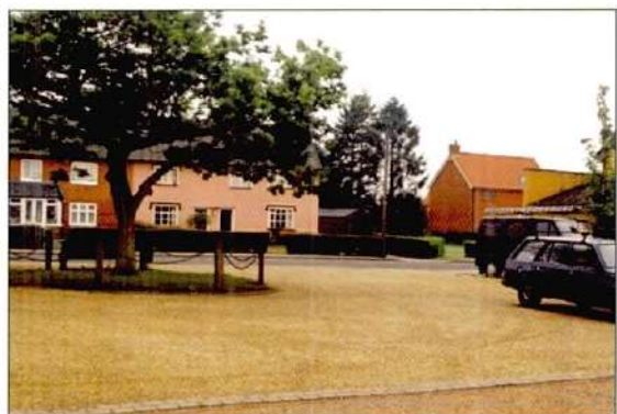
This double dressing at The Square in Dennington has worn well
