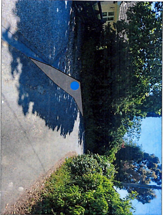
② Edge of carriageway to be tarmaced up to edge of highways boundary, Edging kerb to be installed at edge of tarmac
