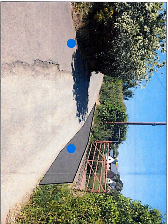
③ Edge of carriageway to be tarmaced up to edge of highways boundary, Edging kerb to be installed at edge of tarmac
