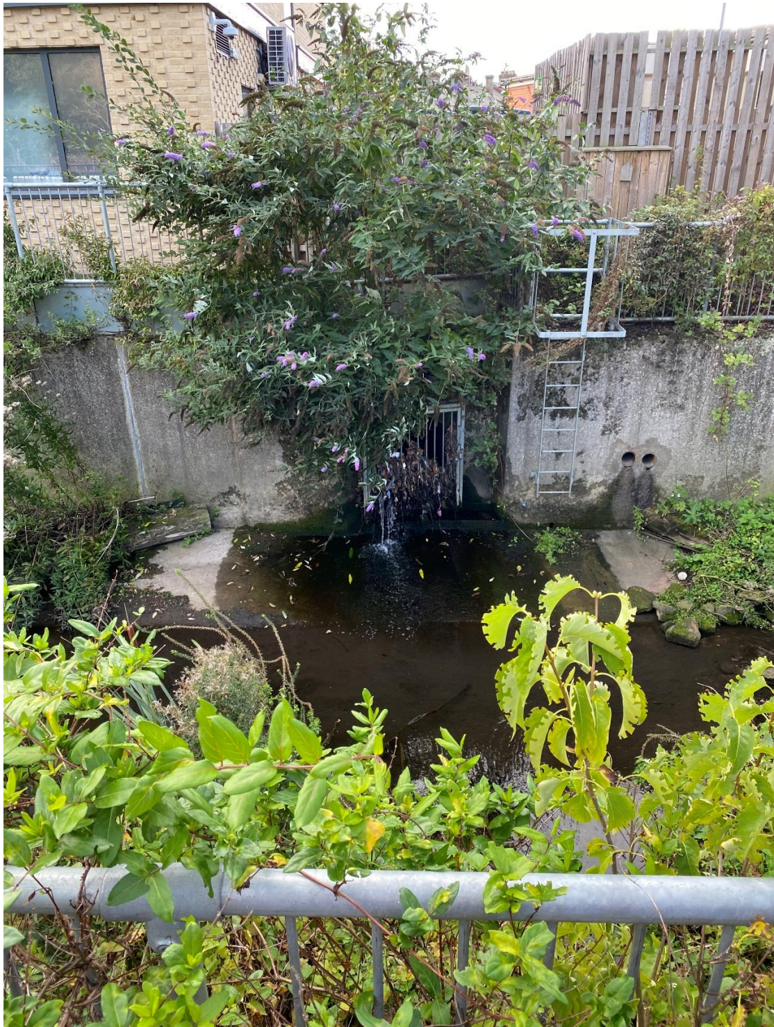
Image 1: Partially blocked outlet pipe from Anglian Water Assets into the river Lark.
