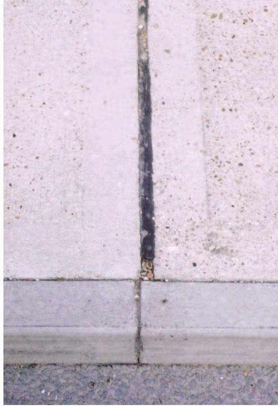
Timber board to form expansion joints is preferable to the use of mastic
