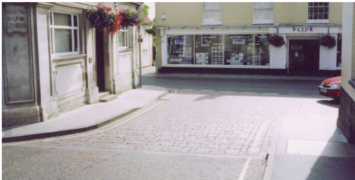
Concrete setts used at a road junction in the centre of the Saxmundham Conservation Area
