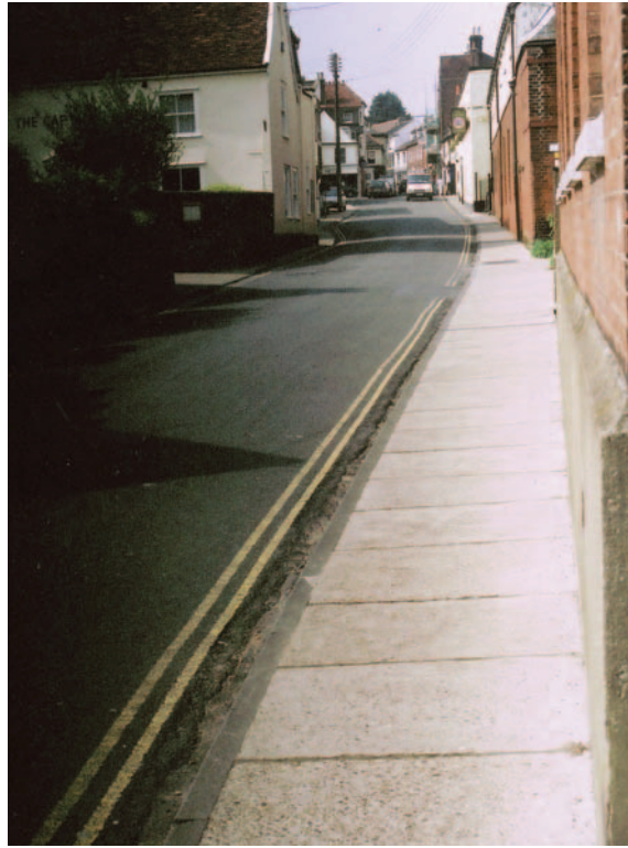
Newly laid exposed aggregate in situ concrete footway in Woodbridge
