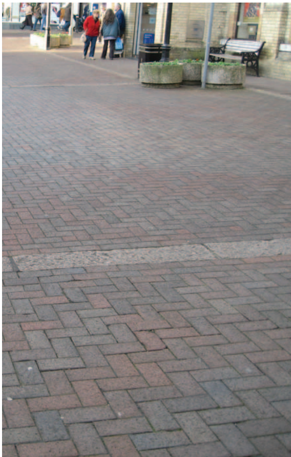
Large areas of rectangular block paviors should be avoided in historic areas
