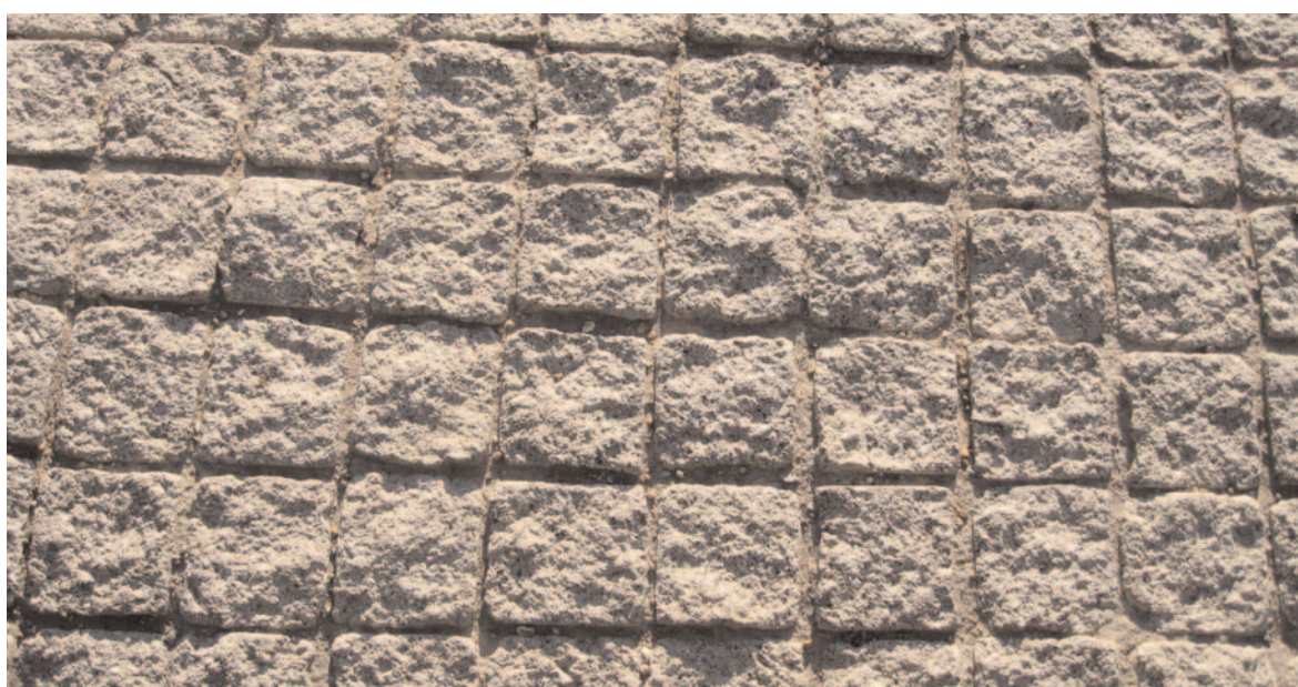
Concrete setts designed to replicate cropped granite cubes
