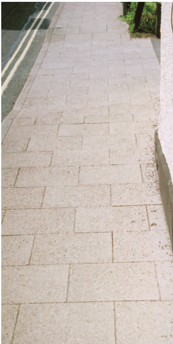
A well laid footway using concrete slabs with an exposed pink granite aggregate (Woodbridge)
