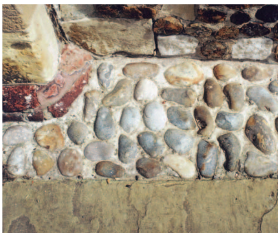
Cobbles neatly laid between an historic building and a riven Yorkstone footway
