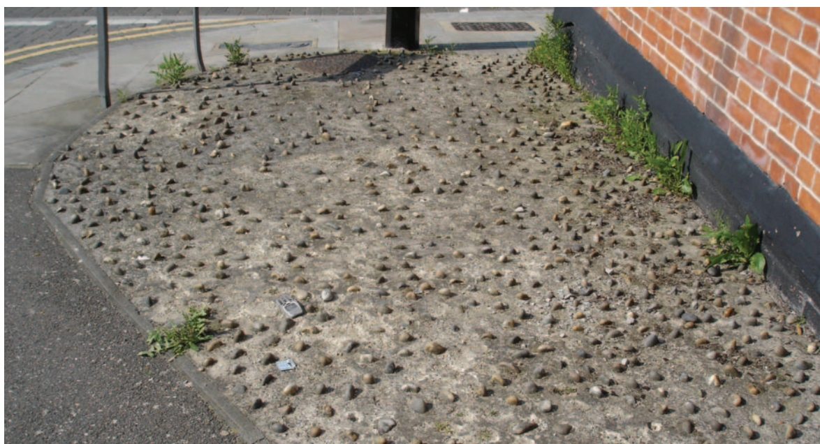
Examples of poorly laid cobbles
