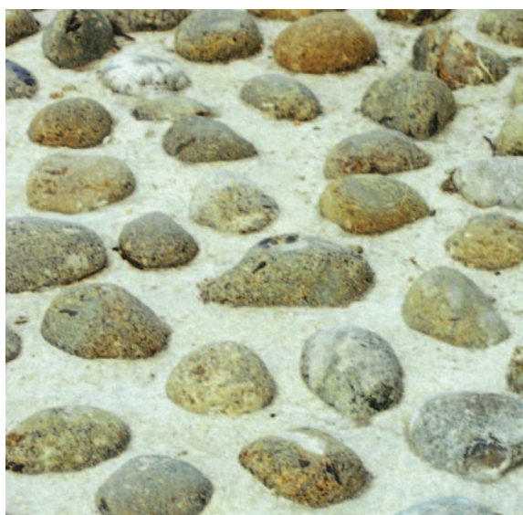
Examples of poorly laid cobbles
