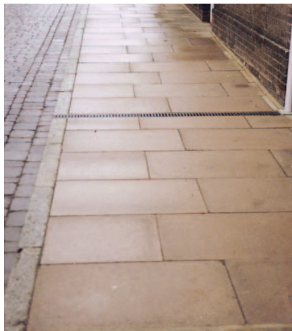
Right: New rectangular concrete paving slabs laid in Bury St Edmunds
