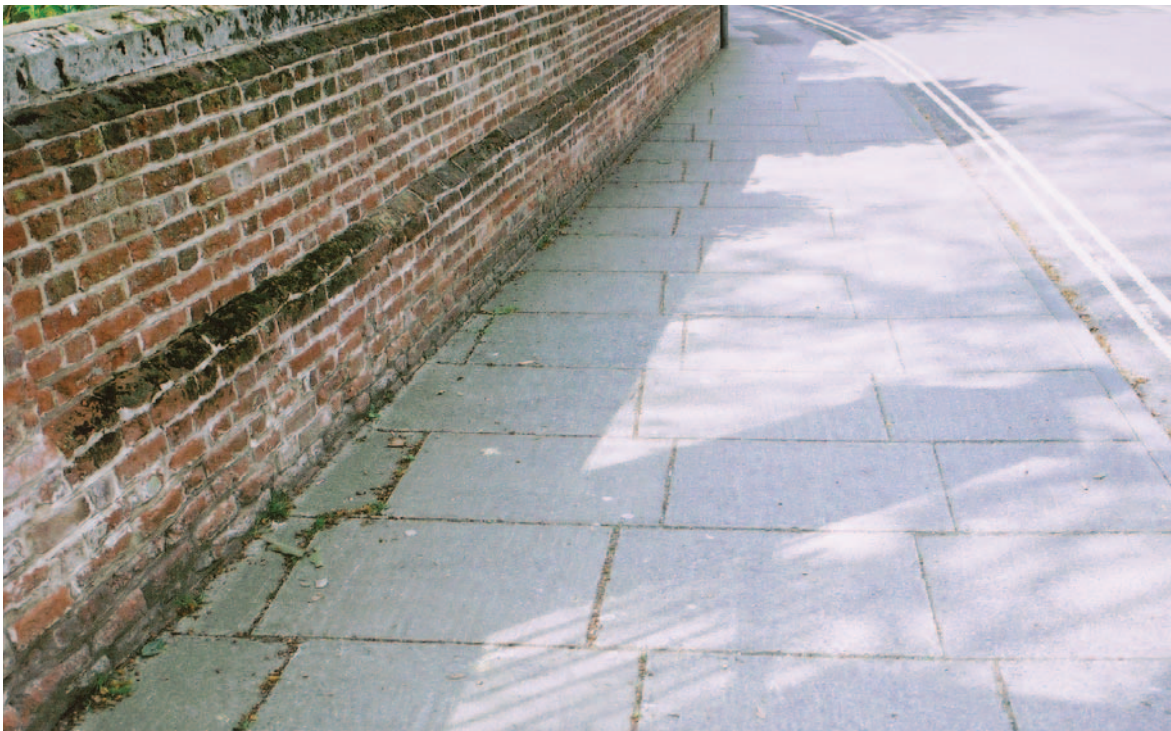
Above: Old concrete paving slabs in Woodbridge
