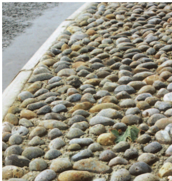
Large cobbles can be used to discourage use by pedestrians
