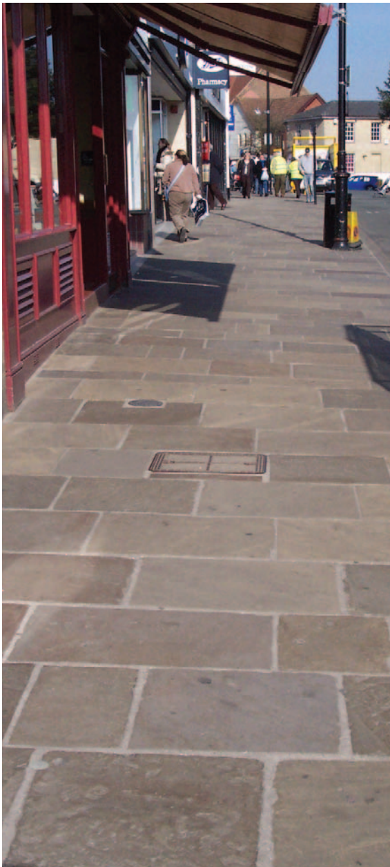
A good example of reclaimed Yorkstone laid in Sudbury
