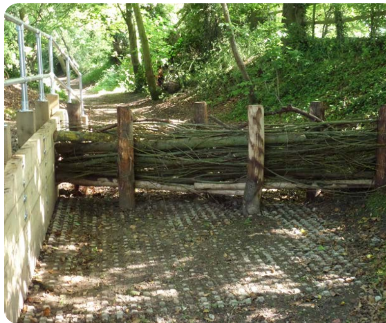
Natural Flood Management – leaky dam.
