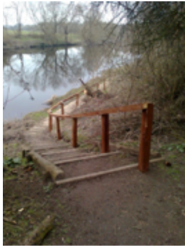
New stepped path down to the River Tees
