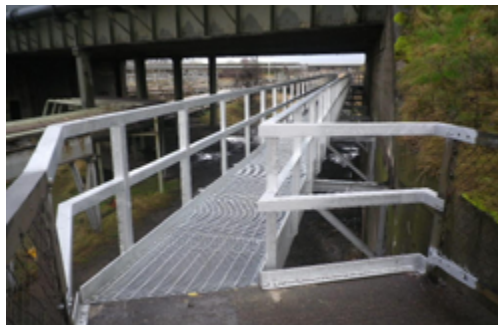
Wilton Steel Works – new Tata Steel Bridge on Teesdale Way in Redcar and Cleveland Borough
