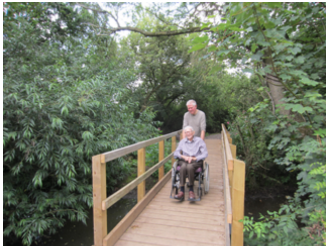
Bridge after improvements
