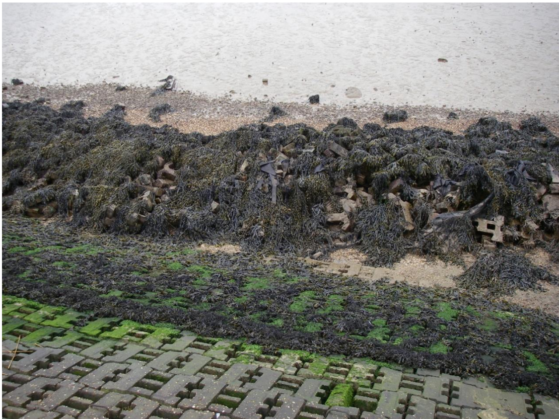
A low energy attenuation/saltings protection bund constructed from Ankalok remnants, this can be found along the Hazlewood frontage of the Alde Estuary.
