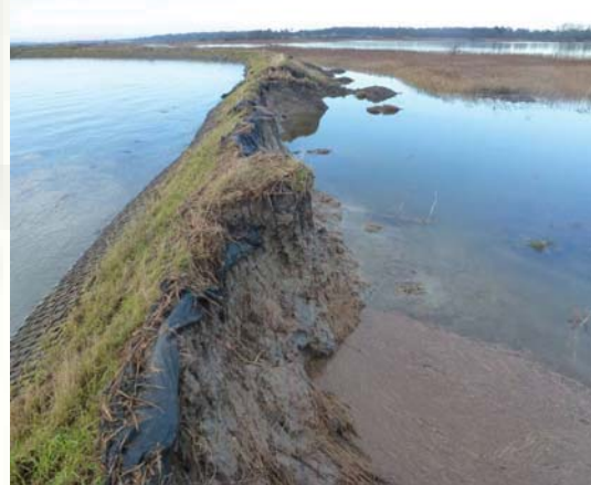
Embankment at Cattawade Marsh after overtopping
