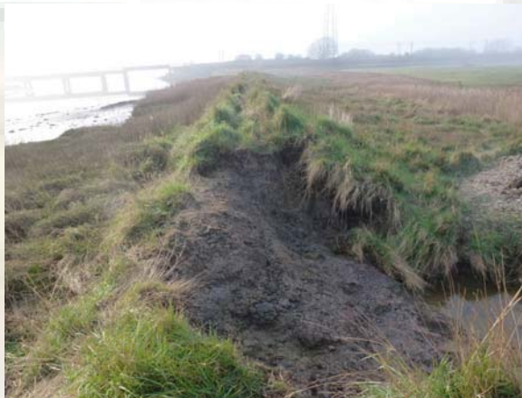
Embankment at Cattawade Marsh after overtopping
