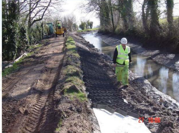
An example of Defencell in use on British Waterways projects
