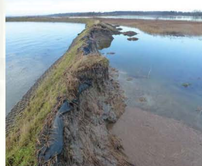
Embankment at Cattawade Marsh after overtopping
