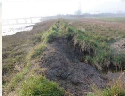
Embankment at Cattawade Marsh after overtopping
