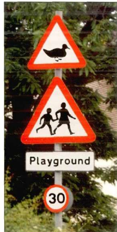
Three signs on one pole without a backing plate
