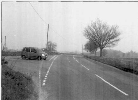
The grass verges were extended at this junction improvement at Playford Corner
