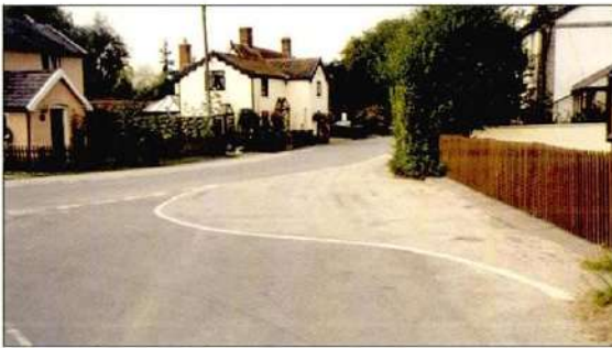
Build-outs using surface dressing and granite setts are a simple and effective measure
