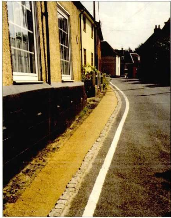
Build-outs using surface dressing and granite setts are a simple and effective measure
