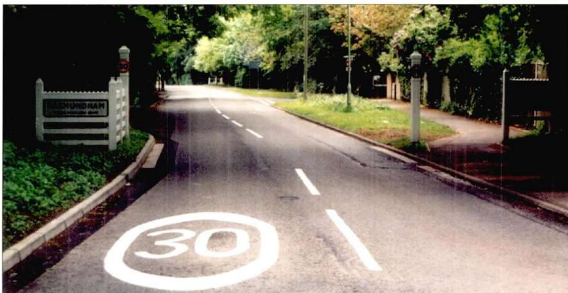
This gateway reflects the character of a traditional toll gate which existed previously nearby
