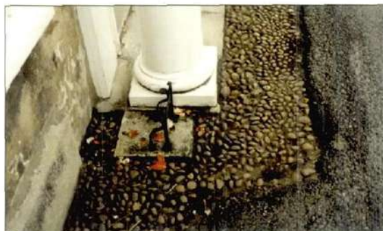
Traditionally laid cobbles
