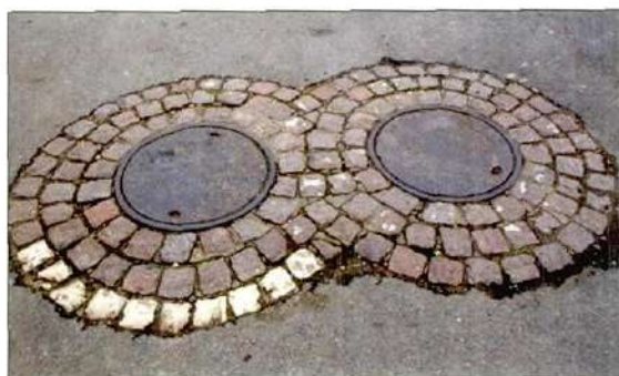
Pink granite setts around manhole covers
