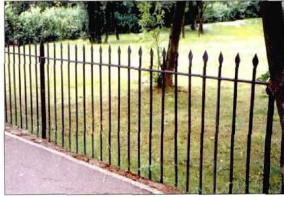
Simple metal railings
