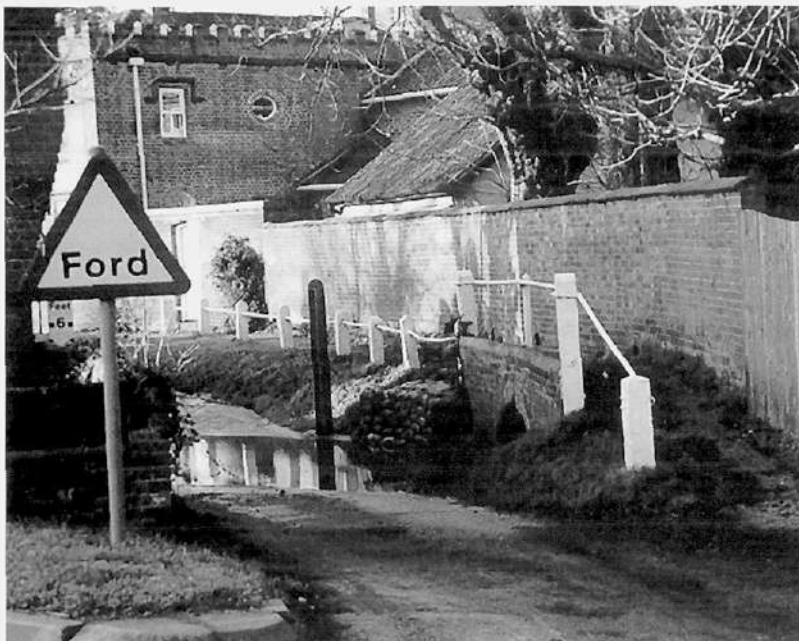
White painted concrete posts and metal rails have been traditionally used in the County as guard rails on bridges, alongside streams etc. This example is in Grundisburgh
