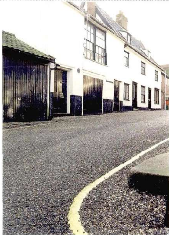
Where yellow lines are absolutely necessary conservation grade lines should be used
