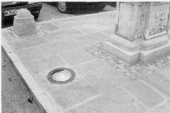
Flush lights within the paving highlight the Obelisk in Chequer Square, Bury St Edmunds
