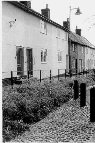
Wooden posts and plain metal post and rails are appropriate to the character of Ixworth
