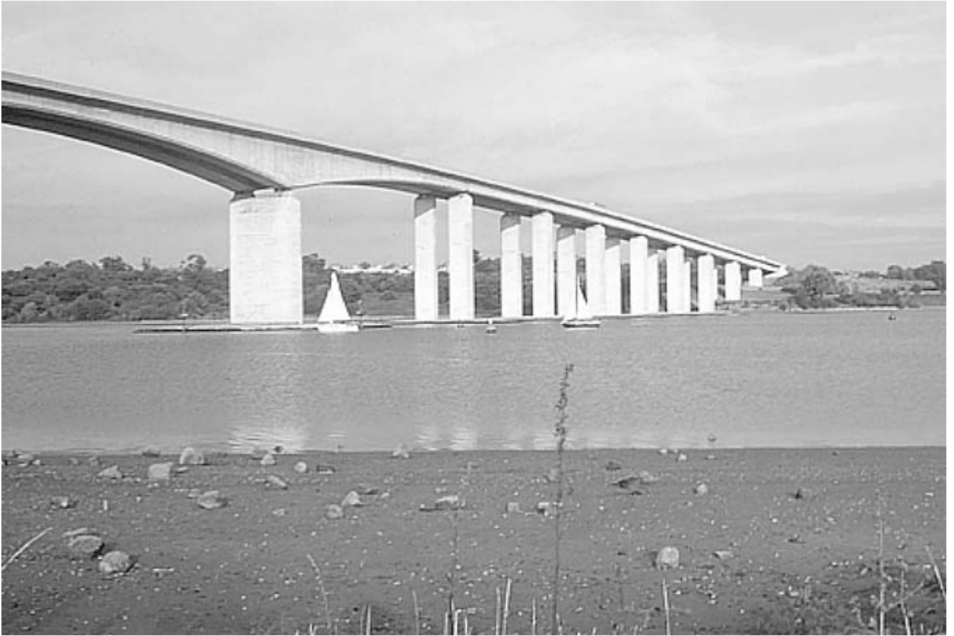
Orwell Bridge, Ipswich
