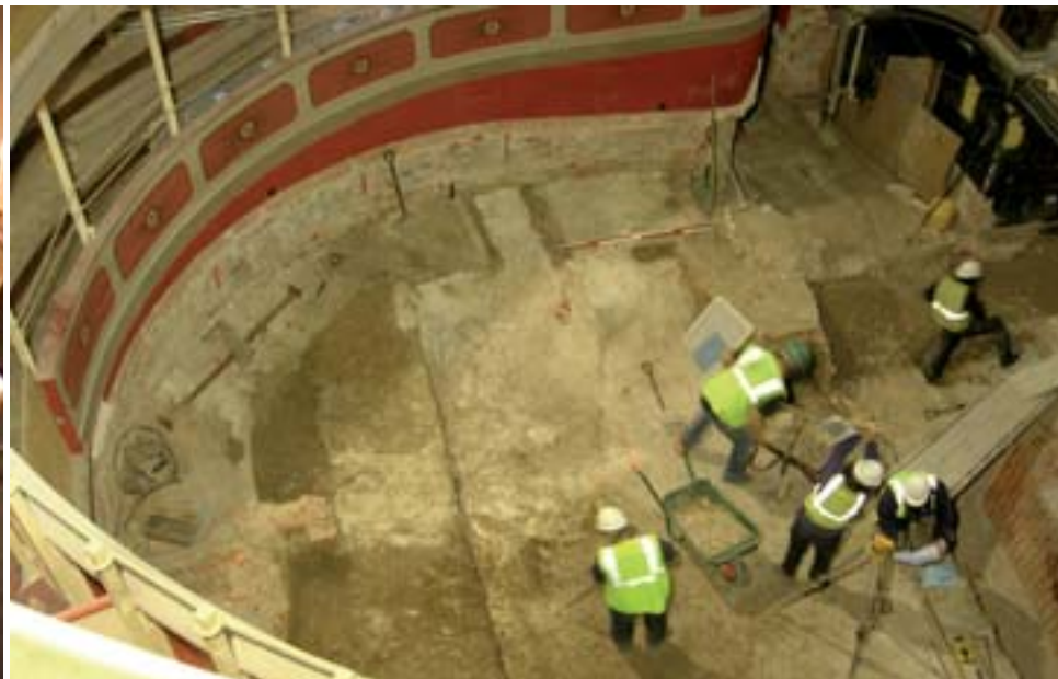
Excavations in the auditorium of The Theatre Royal, Bury St Edmunds
